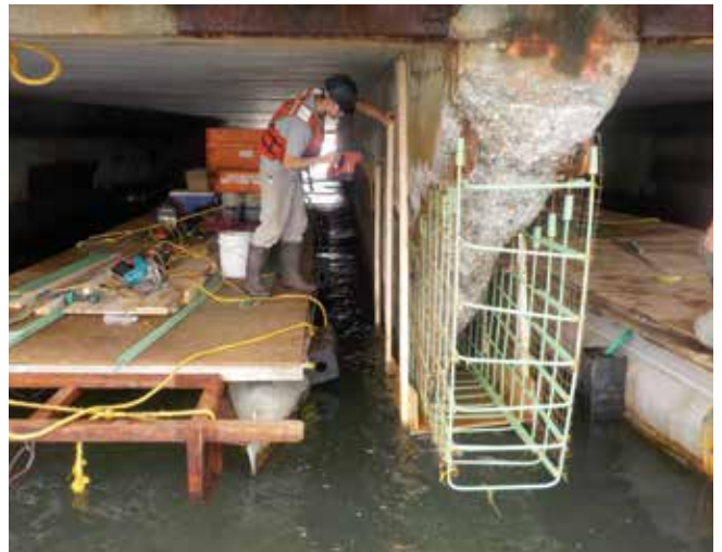
Fig. 4: The installation of a wooden form to help create the right taper of the girder bottom
