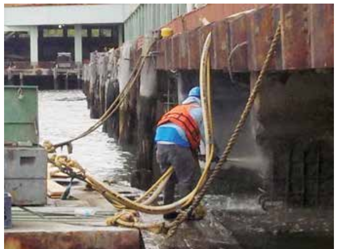
Fig. 5: Eastco's ACI Certified Nozzleman applying shotcrete
