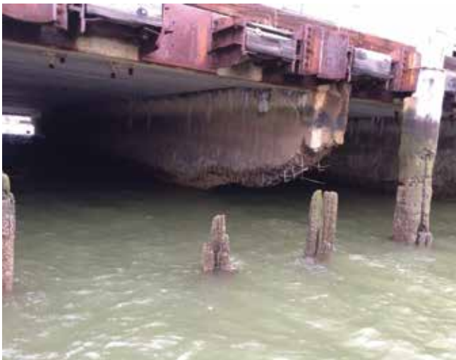
Fig. 1: An example of a moderate girder repair
