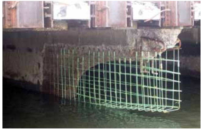
Fig. 3: A reinforcing bar cage using reinforcing bar couplers
