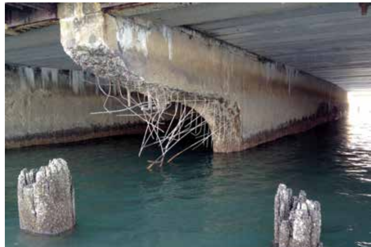
Fig. 2: An example of a severe girder repair
